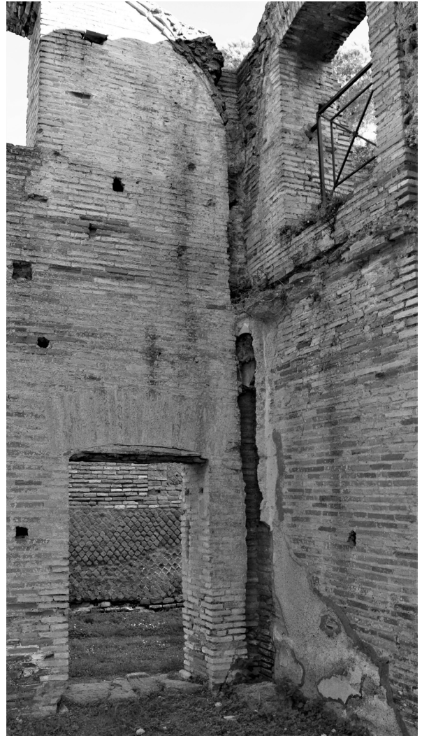
Figure 1.6: Examples of a down-drain extending above the ground floor in the Caseggiato dell Serapide (III, x, 3), which still contains a circular ceramic pipe within the masonry shaft.
